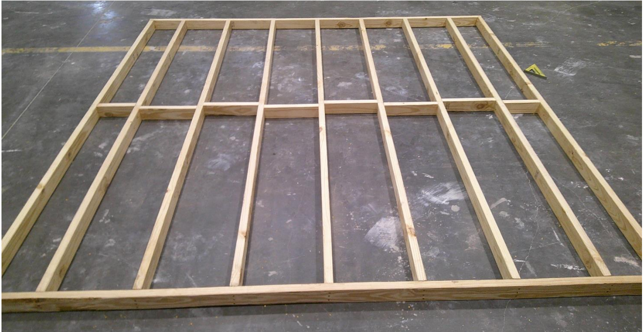
Photo No. 1 Completed framing of base wall
