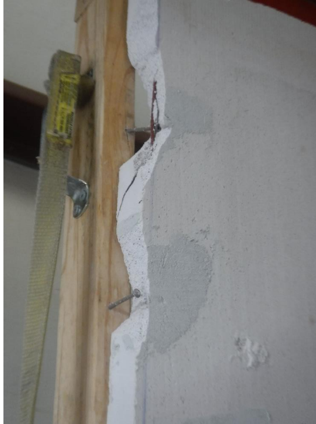
Photo No. 17 Example 2 of Racking Test Failure (Wood Frame)
